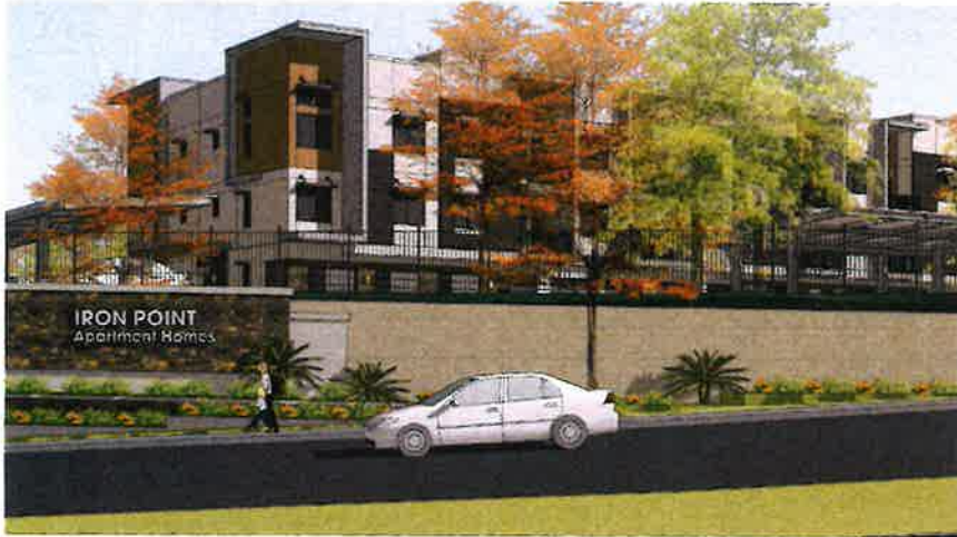
NORTH VIEW OF LOT 6 FROM IRON POINT RD. CORNER
