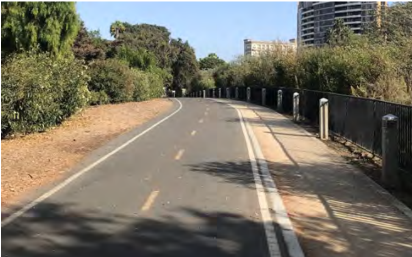
A soft-surface shoulder alongside a shared use path provides additional space for path users, particularly runners or others who prefer natural surface paths.
