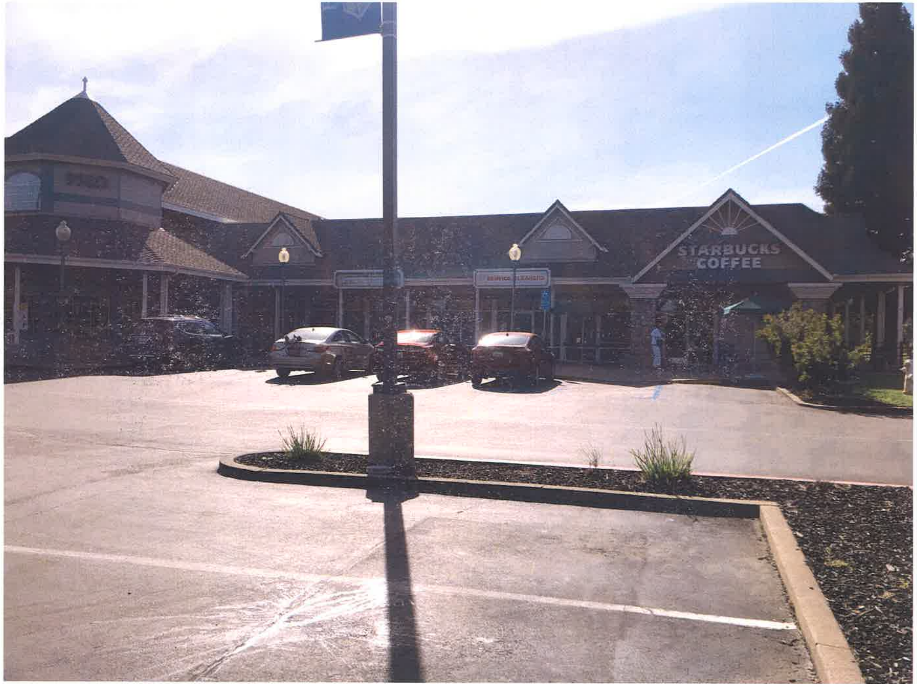
Parking Lot View of Store
