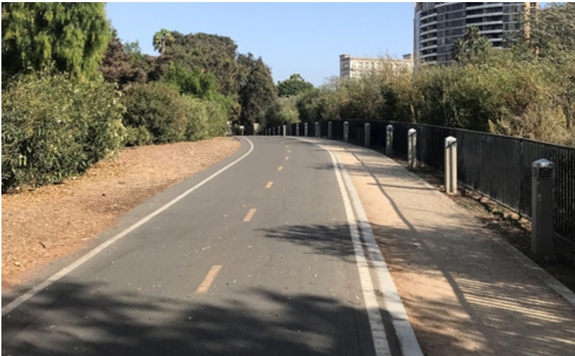
A soft-surface shoulder alongside a shared use path provides additional space for path users, particularly runners or others who prefer natural surface paths.
