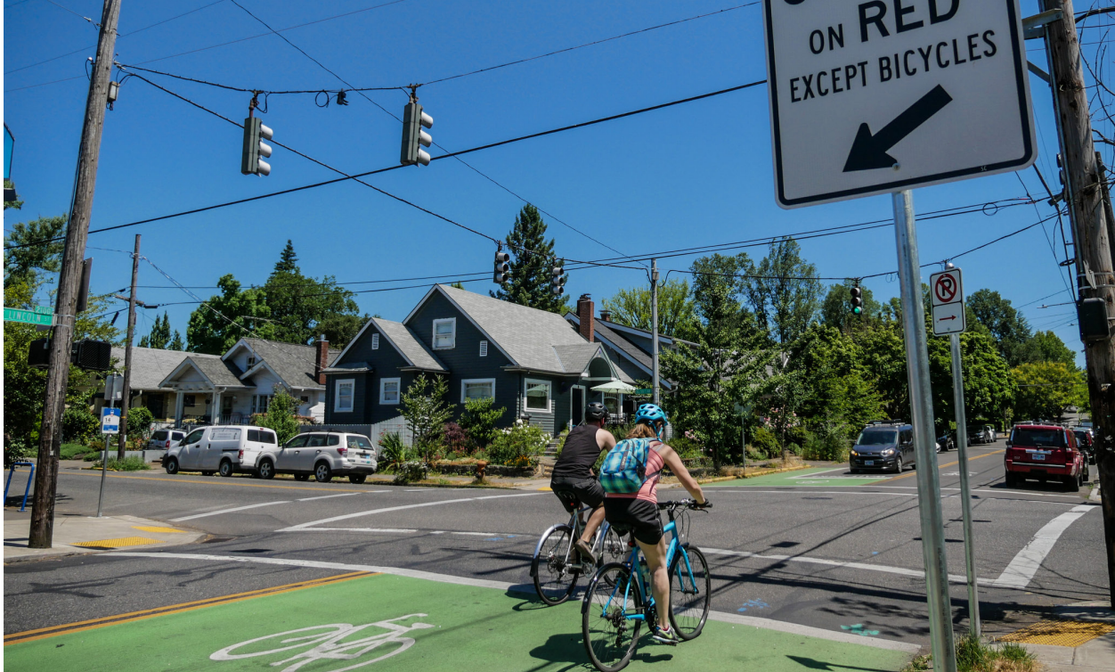
A bike box allows for bicyclists to wait in front of queuing traffic, providing high visibility and a head start over motor vehicle traffic.
