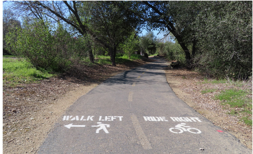
Pavement signage further emphasizes that the path is bi-directional and shared among a variety of users. While this does not create additional space, it provides reminders of path etiquette along the length of the path.
