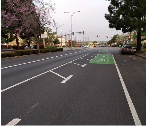
Buffered bike lane transitions into dotted green and white lane markings to indicate conflict point
