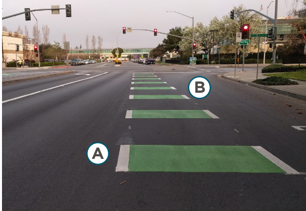
Green colored conflict striping indicates the path of travel of people on bicycles, and alerts people intending to turn across the bike lane to yield when bicyclists are present.
