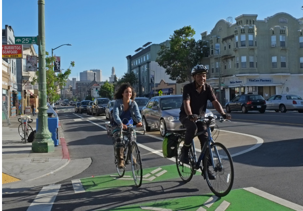
Parked cars serve as a barrier between bicyclists and the vehicle lane. Barriers could also include flexible posts, bollards, planters, or other design elements Source: Bike East Bay.
