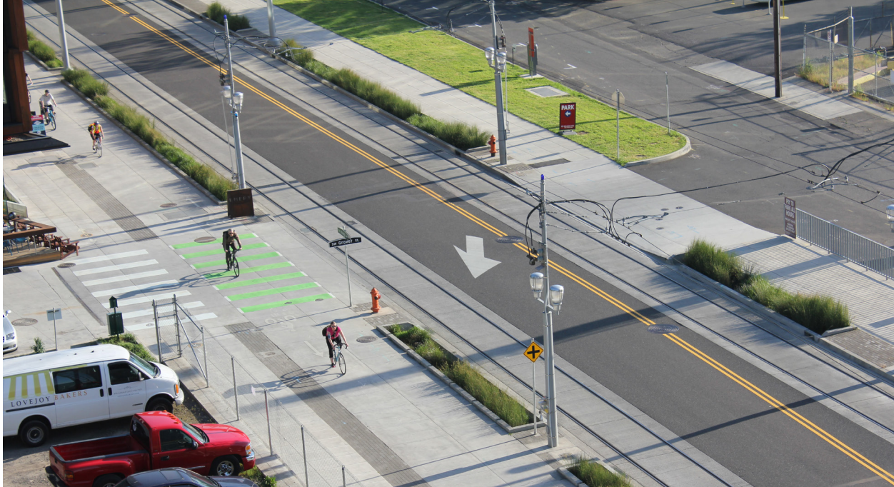
Intersection crossing markings can be used at high volume driveway and minor street crossings, as illustrated above.
