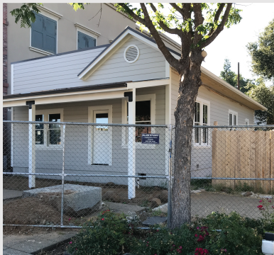
Current condition of building.
