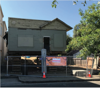
Building raised for its new foundation.
