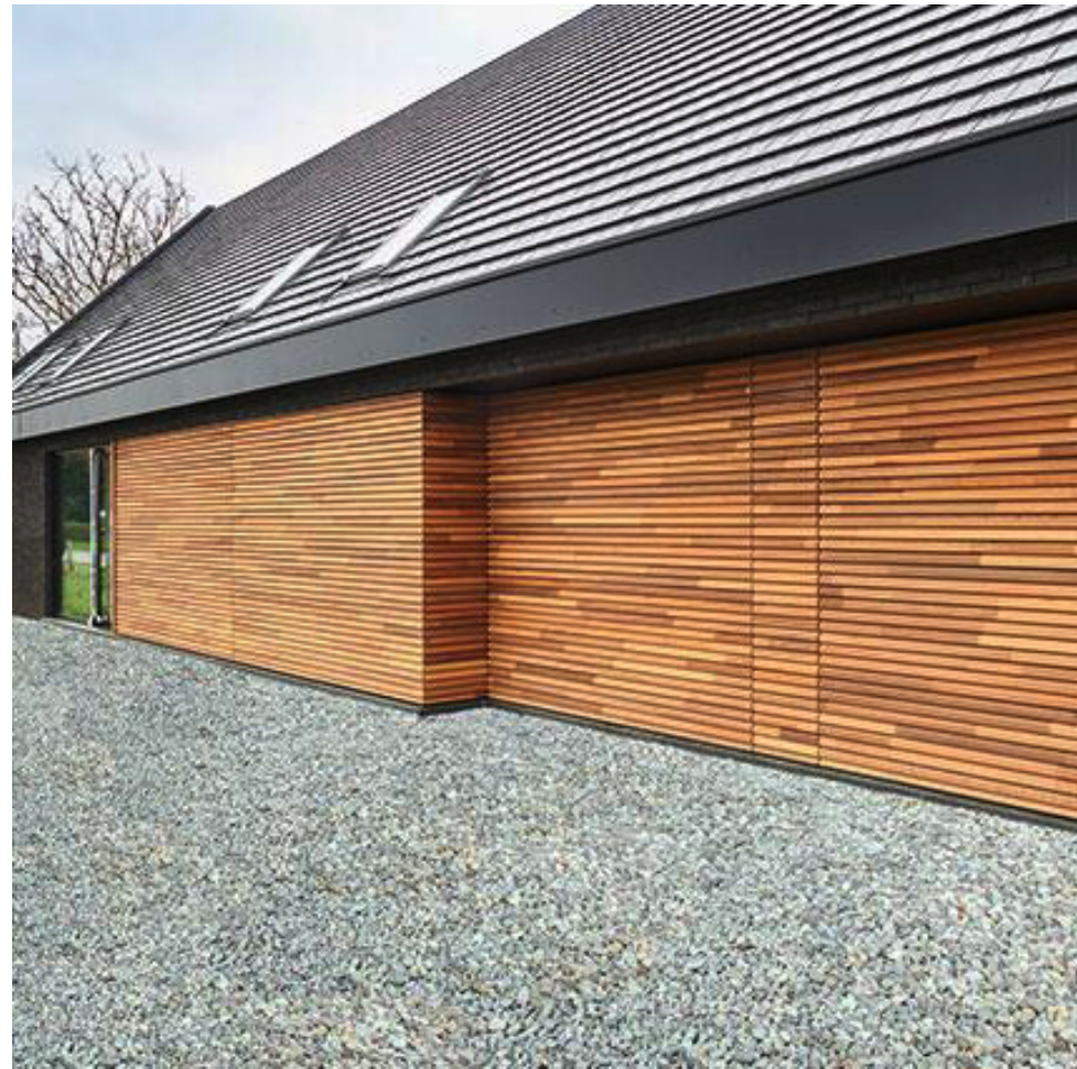
WOODEN GARAGE DOOR INTEGRATED WITH THE FACADE CLADDING (FLUSH-FITTING)
