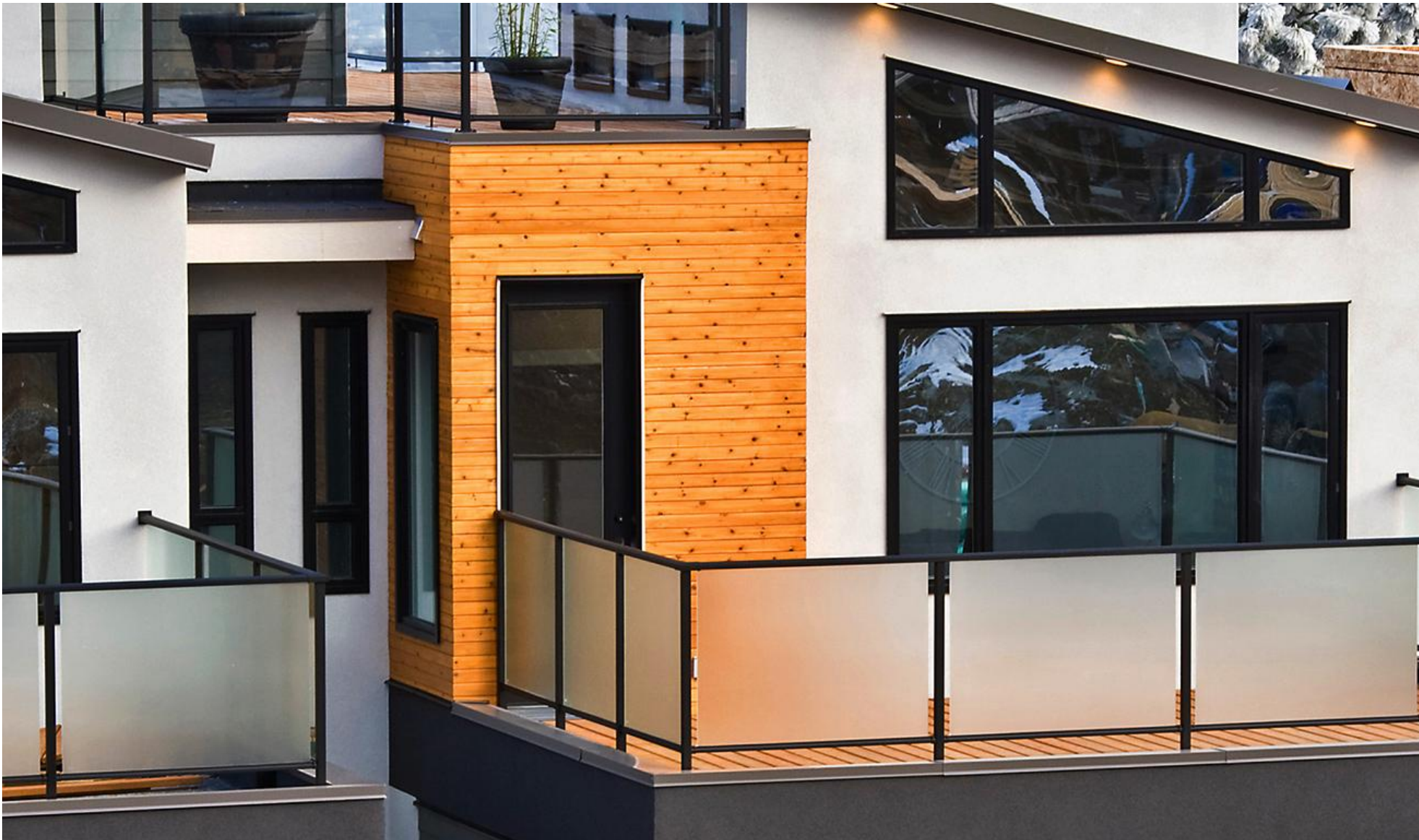
WINDOWS: BY ALL WEATHER WINDOW. APEX ALLOY 9950 FRAME: ALUMINUM CLAD PVC. COLOR: BLACK
