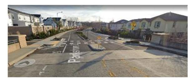
Crossing distance is approximately 38' ramp to ramp with a center island, appropriate signage. Striping on the bridge is showing signs of wear but the crosswalks, signs, and pedestrians are highly visible in approach to the intersections.
