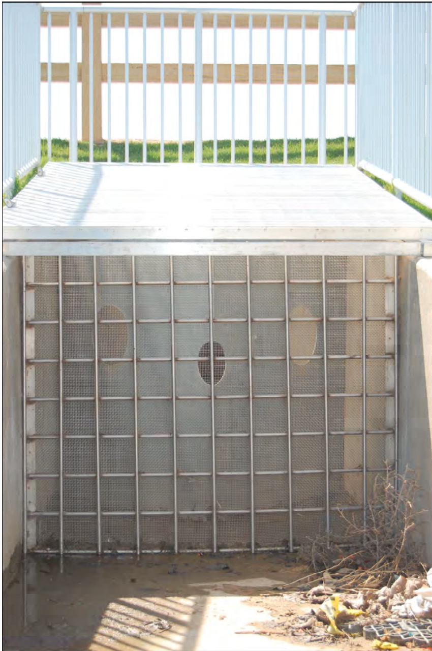
Figure 6 - Flow duration control outlet structure. Notice different sized orifice located at varying elevations to mimic pre-project flow rates and duration. (Photograph taken by C. Bowles, Hitachi Redevelopment, City of San Jose, 2009).
