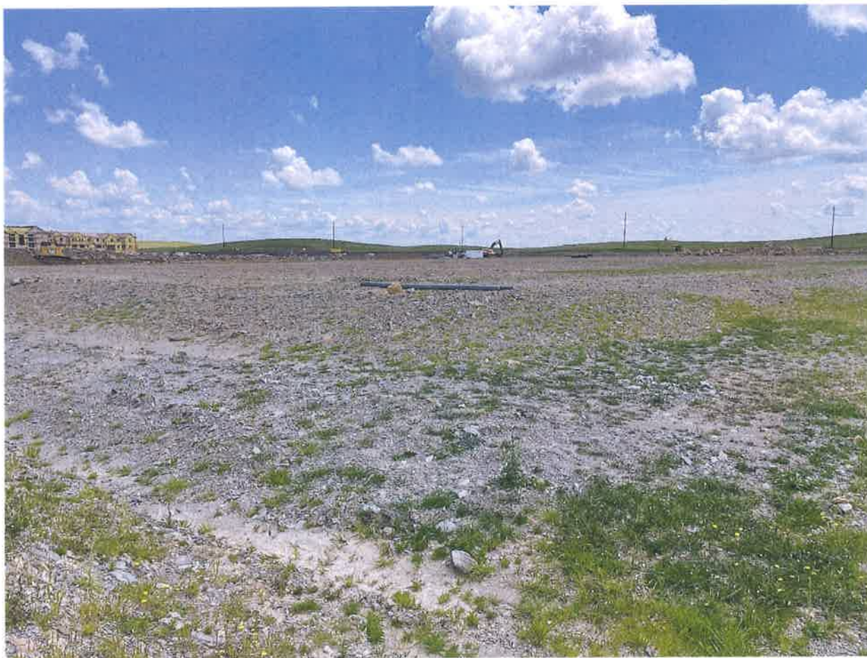
FIGURE 2: PHOTOGRAPH OF PROJECT SITE
