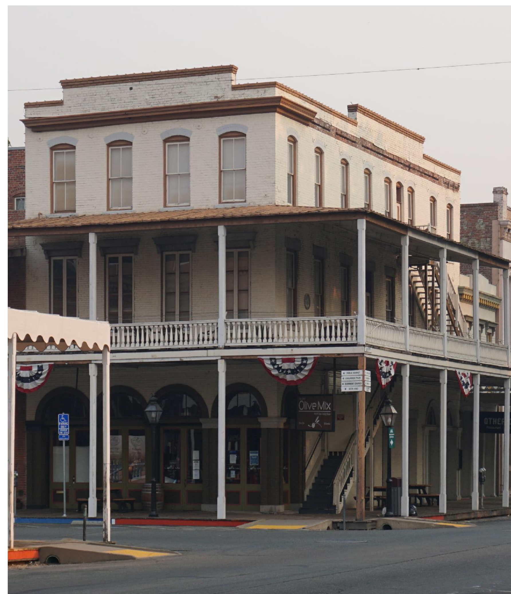
REFERENCE - 3 STORY BLDG. - OLD SACRAMENTO
