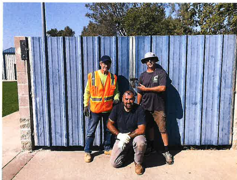
Upper Livermore Trash Enclosure Repair
