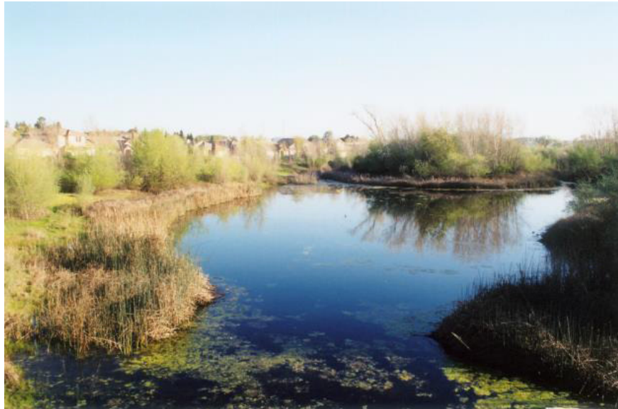
The detention basins may hold water during and immediately after each storm.
