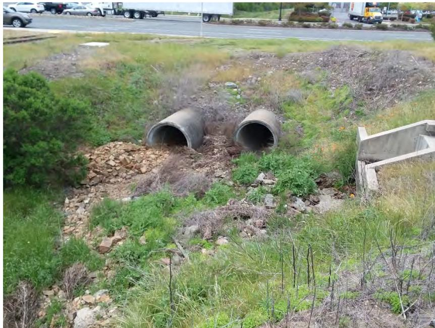
Photo 5: Culvert structures direct hydrologic flows into the wetlands underneath roadway at Folsom/Placerville Rail Trail site.
