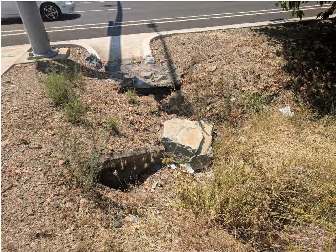
Photo 18. Damaged drainage feature at E Bidwell St and College Pkwy intersection
