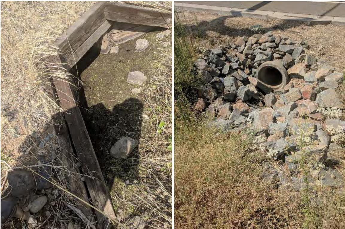
Photo 10. Culvert inlet west of railroad track (left); culvert outlet east of railroad track, facing southwest (right)
