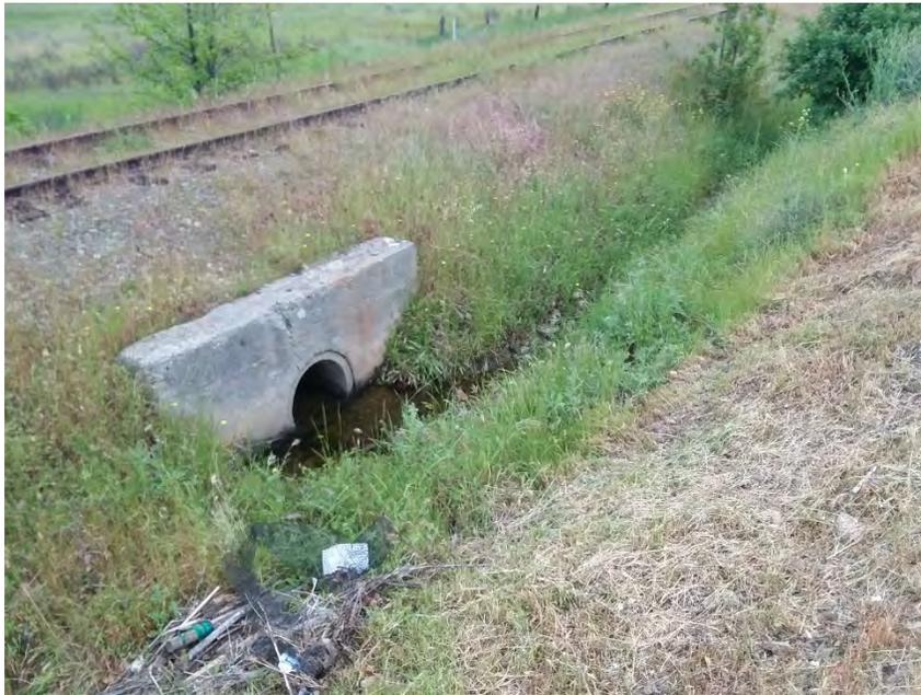
Photo 6: Culvert structure allows hydrologic flows into wetland at Folsom/Placerville Rail Trail site.
