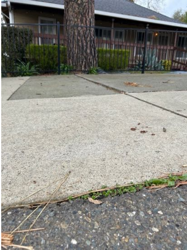
Left: Lifting from roots is causing damage to a permanent structure; driveway/sidewalk.
