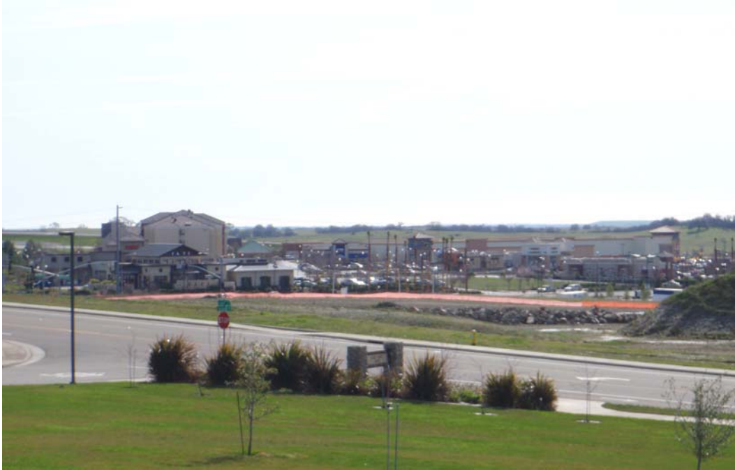
Viewpoint 13: View from Handy Family Park, located within the City of Folsom. The middleground contains a view of the central lowlands and oak woodlands portion of the SPA. The Coast Range is located in the background. (AECOM 2009)
