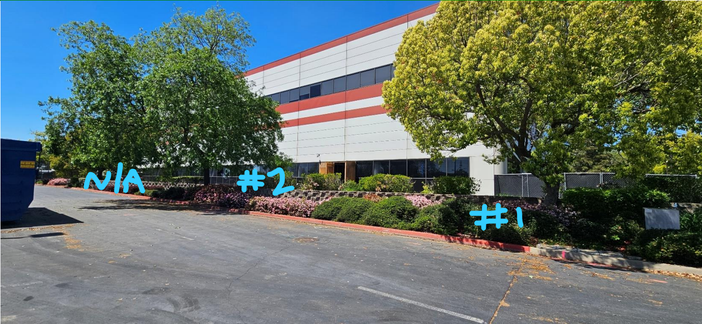
Site view of trees in construction area
