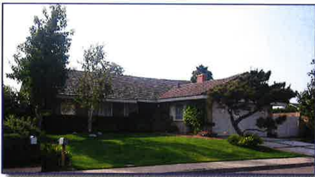
Example of California Ranch Architecture
