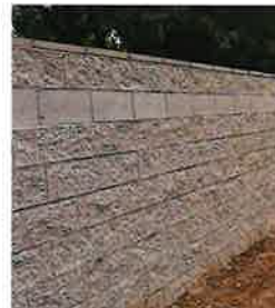
6' HIGH MASONRY WALL
