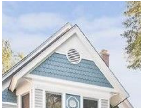
Fish scale shingles with vent at end of forward-facing gable
