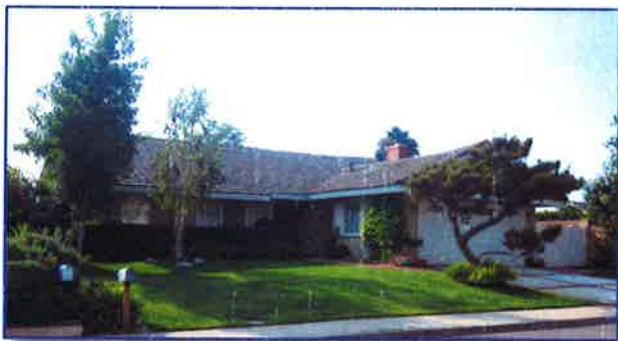
Example of California Ranch Architecture
