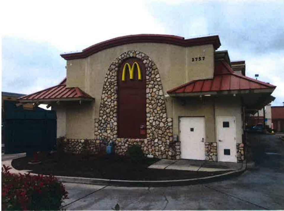
Photo -7- Rear Elevation at E. Bidwell St. side
