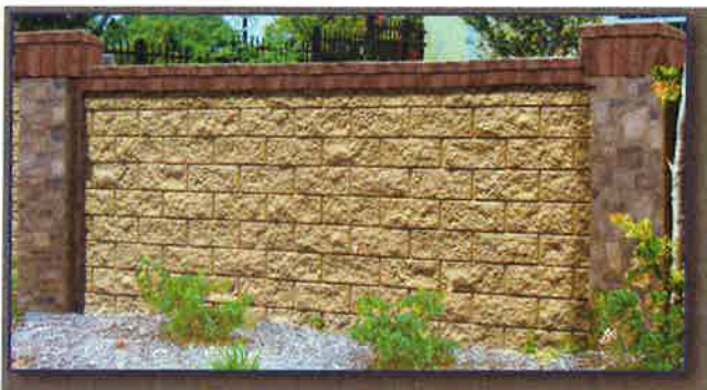
Community Wall and Pilaster
