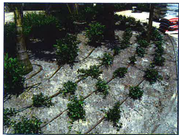
Example of Drip Irrigation Before Mulch
