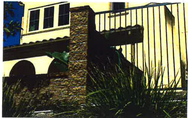
Prefabricated Tubular Steel Fence with Pilaster Condition Pilaster: Split face Block with Brick Cap Block Color: Harvest (or equal) available through Angelus Block Paint: Sherwin Williams SW7705 Wheat Penny Brick: Belden Brick- Jumbo Polar White Clear A (Sugar creek Plant 3), available through Thompson Building Supply Grout: CBP #384 Camel Metal Color: Powder Coated- Sherwin Williams SW7020 Black Fox
