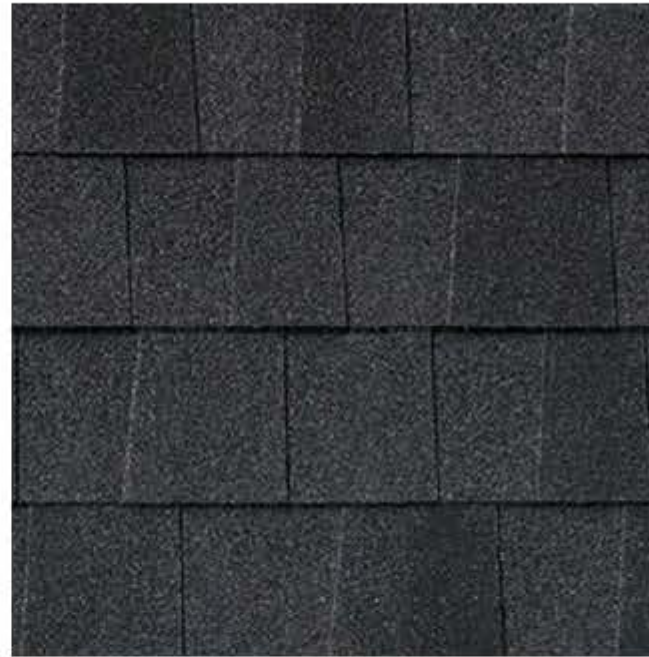
ASPALT SHINGLE ROOF
