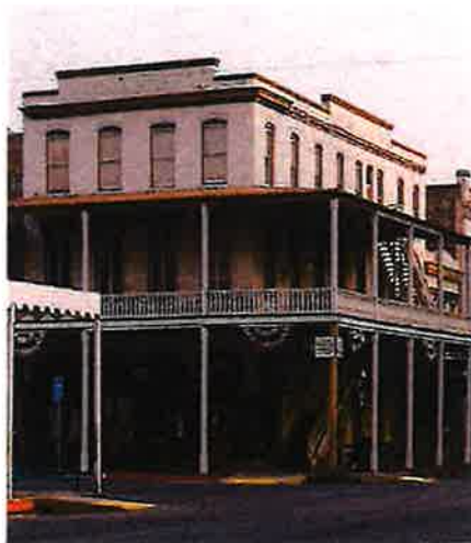
REFERENCE - 3 STORY BLDG. - OLD SACRAMENTO
