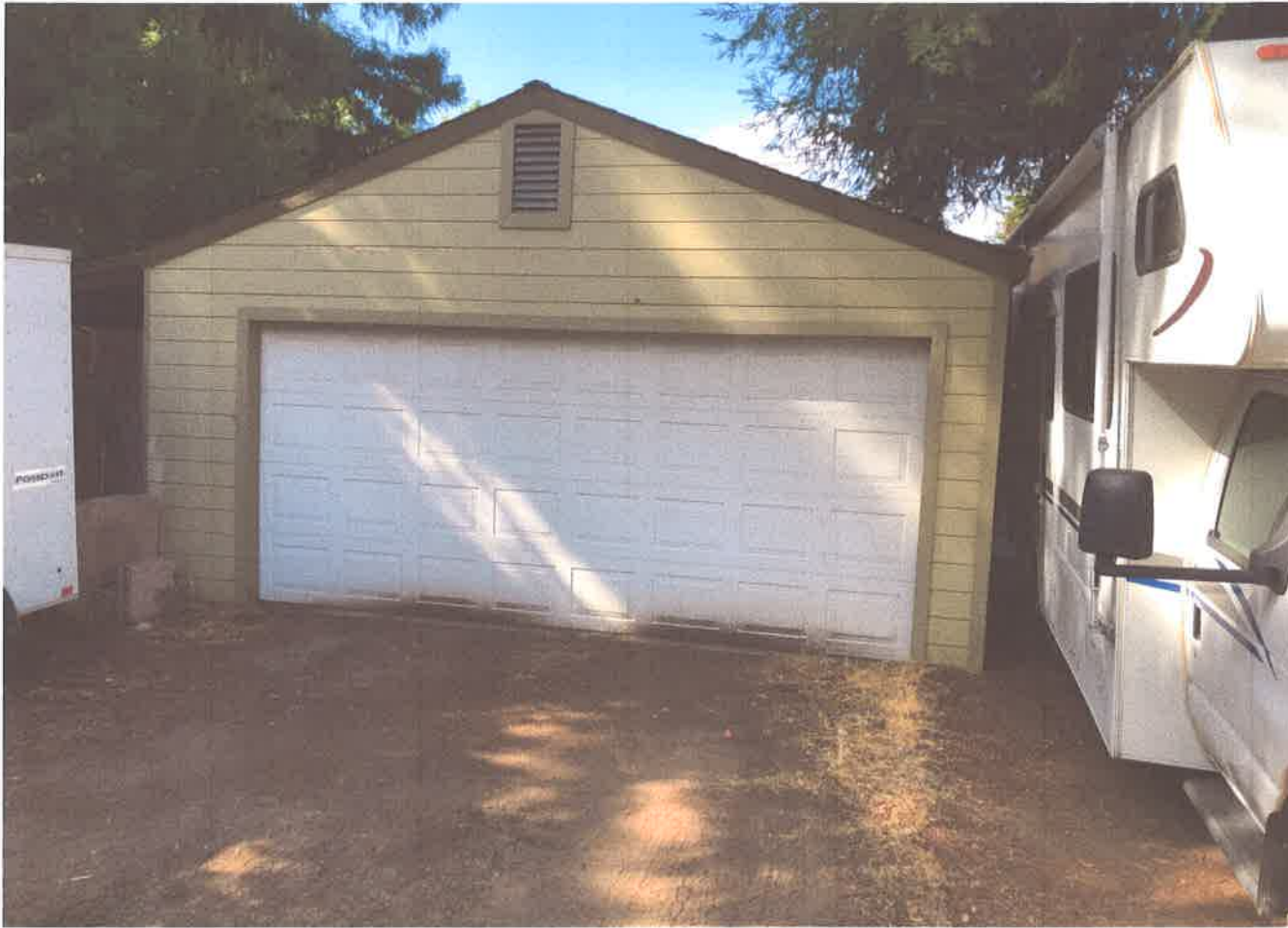
NE SIDE ALLEY VIEW
