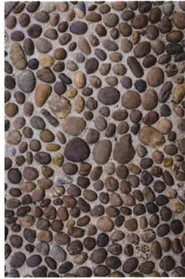
COBBLE AT COLUMN BASES
