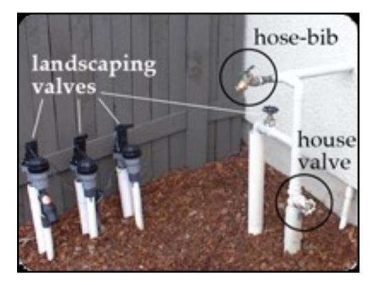
Inspect areas around the valves or valve manifold for leaks and/or pooling water.
