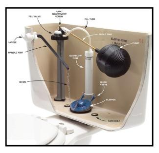
Make sure the water refill level is set properly and does not rise over the top of the overflow tube.
