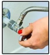
Before replacing any parts on your toilet, be sure to follow the part manufacturer's installation instructions and turn off the water supply valve to the tank (usually found on the wall behind the toilet). When turning off the water supply valve to the toilet, simply turn the knob until it is snug but not tight to prevent it from breaking off or coming loose.
