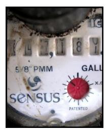
Check the flow indicator again. If it has stopped turning, you have a leak in your irrigation system.
