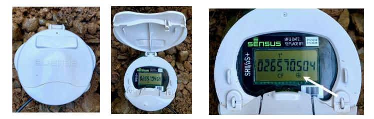
Digital meters have a lid which must be opened to access the face. The reading will only be visible for a short time. It will shut off after a moment to preserve battery strength. If this happens shut the lid securely, wait a moment and open it, the reading should be visible once again.
