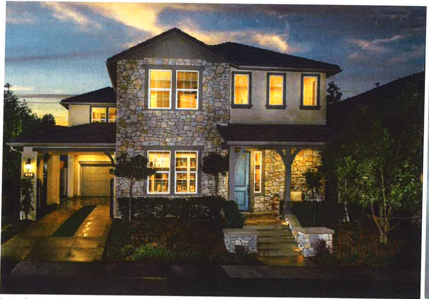
Porte Cochere with Garage at Rear of House
