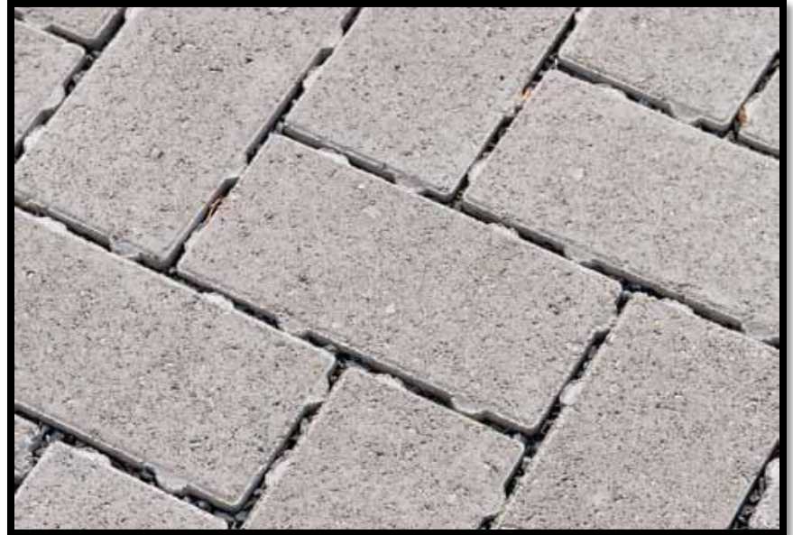
Interlocking concrete pavers w/spacers
