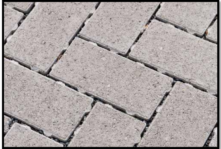
Interlocking concrete pavers w/spacers
