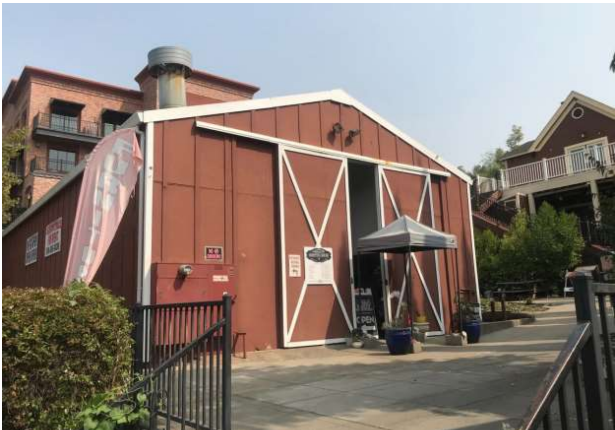
FIGURE 4: COMMERCIAL BUILDING AT 608 ½ SUTTER STREET
